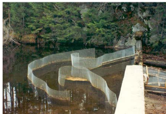
Deflector and collector screens in front of an inclined screen trap
