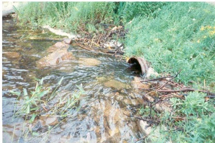
Small diameter culvert drain pipe
