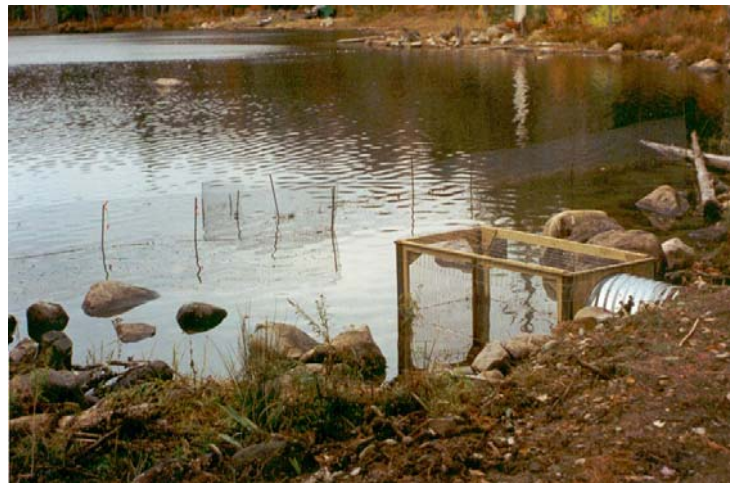
Culvert-box style outlet barrier
