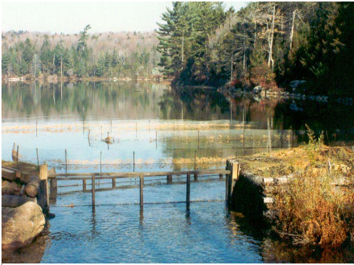
Screen-weir outlet barrier system with log cribs and keyways
