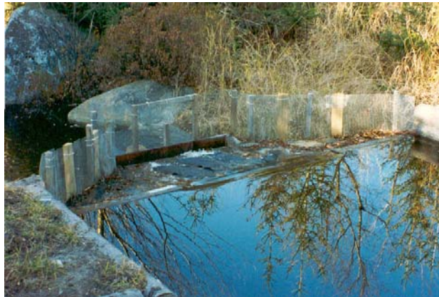
Inclined screen trap
